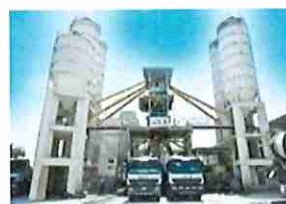
Ready-mix Concrete Plant
