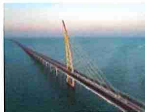
Jaber Al Sabah Bridge
